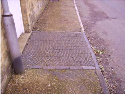
Brick paviours to the footway in Weekley Wood Lane
